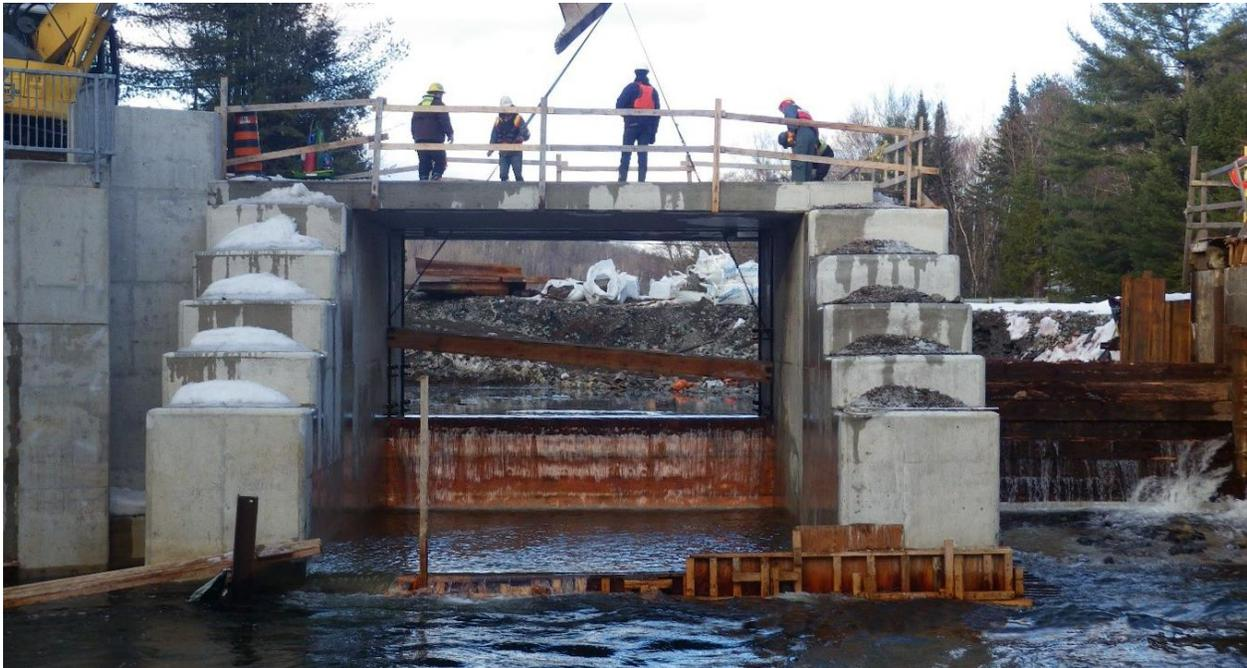
Parks Canada engineers and dam operators on-site to inspect stoplogs being lowered into a brand new sluice at Horseshoe Lake Dam. (February 2018)
